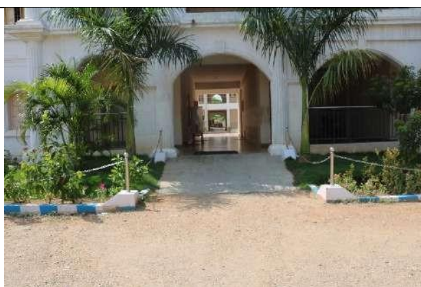
Ramp at Left Side of the Building
