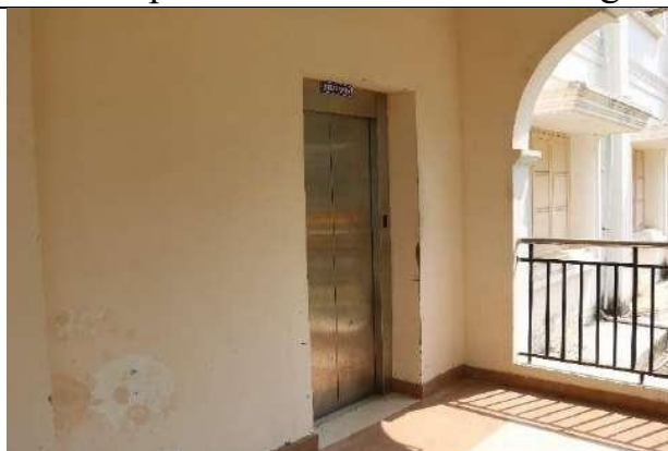
Elevator at Left Side of the Building
