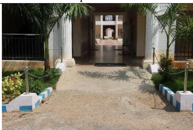
Ramp at Right Side of the Building
